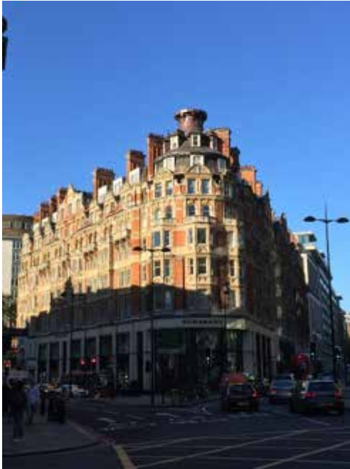
Example of large-scale blocks
