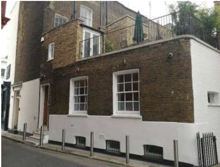
20 Montpelier Street, side & rear elevations
