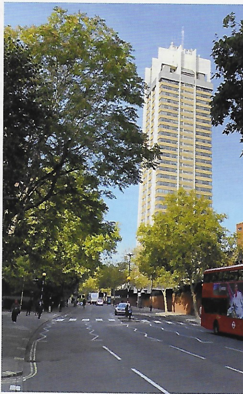
Dangerous pedestrian crossing at Trevor Place/Trevor Street
