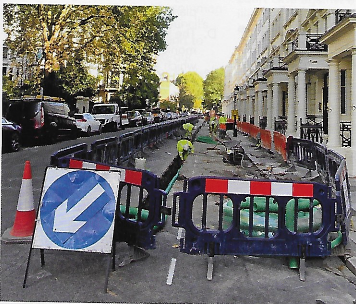
Fibre optic cable works in Ennismore Gardens
